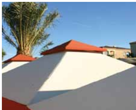
Roof-Top Air Vent
